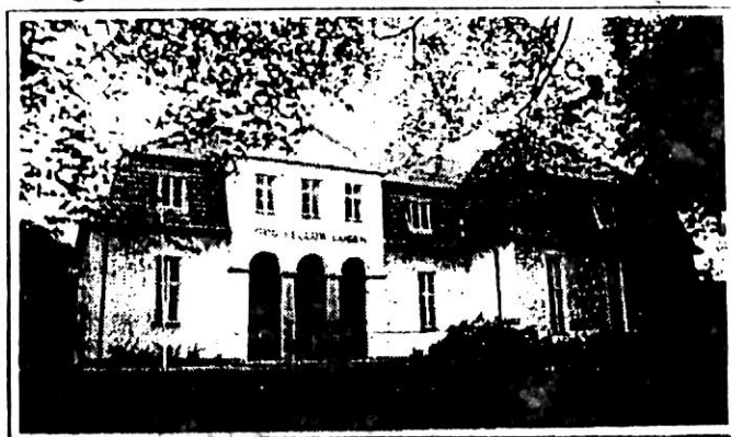
Odd Fellow House, Odense, Denmark
